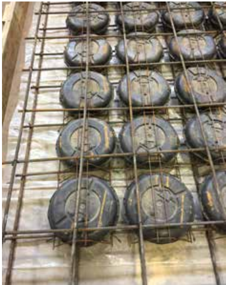
Figure 2. Layout of void formers in test assembly
