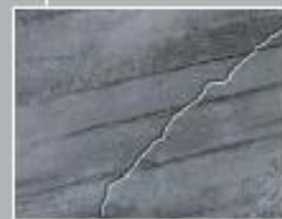
Structural Crack and Void Repair
