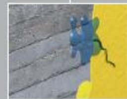
Waterproofing of damaged Membranes
