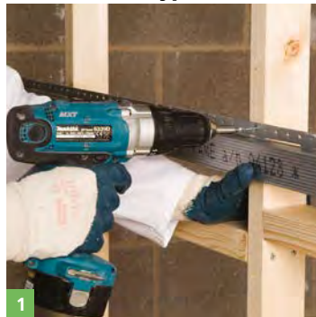
2 Resilient Bar fixed to one side
