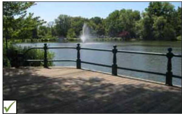
Example of protective barrier where there is a large elevation change, or trail is adjacent to water feature.
