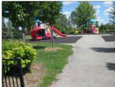
Accessible route connecting to play space.
