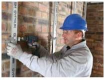
Gypframe Bracket legs are bent forward and each leg fixed to the Gypframe GL1 Lining Channel with Gyproc Wafer Head Drywall Screws.
