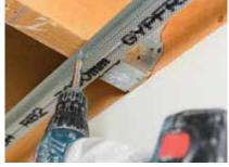
Alternatively, Gypframe RB1 Resilient Bars are fixed through the single fixing flange to the underside of timber joists (at 90° to them) using Gyproc Drywall Screws. The first and last rows of Gypframe RB1 Resilient Bars are located at all wall perimeters.
