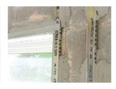
At angles and reveals, Gypframe MF10 Channels are installed close to the corner to provide support. Door and window openings are framed with Gypframe MF10 Channels. At window openings, the channel at the head forms a ground for fixing curtain track. Where a partition abuts, an additional Gypframe MF10 Channel is installed to provide a fixing ground. Board fixing can proceed once the adhesive has fully set.
