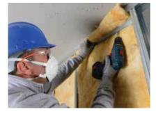
Isover insulation can also be added to the partition cavity for increased acoustic performance.
