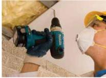
100mm Isover Spacesaver Ready-Cut is laid between joists to rest on the Gypframe RB1 Resilient Bars. The specified ceiling boards are then screw fixed to the Gypframe RB1 Resilient Bars with the correct length Gyproc Drywall Screws to ensure the screws do not contact the timber joists.
