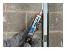
The perimeter of the partition is then sealed on both sides with Gyproc Sealant.
