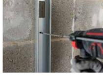
Gypframe 'C' Studs are suitably fixed to abutments in two rows.
