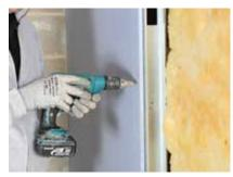
Gyproc plasterboards are then fixed to the Gypframe framework with Gyproc Jack-Point Screws.
