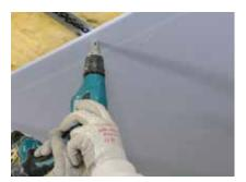
Gyproc plasterboards are fixed to the underside of Gypframe RB1 Resilient Bars with Gyproc Drywall Screws.
