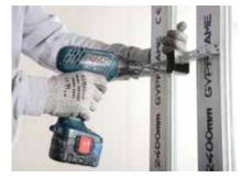
The Gypframe 92 S 10 'C' Studs are then braced together in pairs with either staggered Gypframe GAB3 Acoustic Braces,
