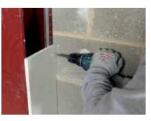
Glasroc F FIRECASE boards are cut to width and fixed to the Gypframe FEA1 Steel Angles with Glasroc F FIRECASE Screws.
