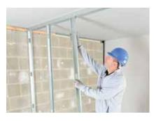
Gypframe 'I' Studs or 'C' Studs are then friction fitted into the Gypframe Channels at required centres.
