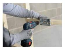
M&E services can be located within the partition cavity before the partition has been boarded. Timber noggings are fixed to support recessed switch boxes / socket outlets.
