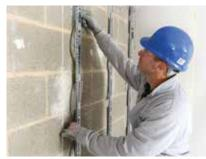
The board edge and centre positions are marked on the wall and dabs of Gyproc Plasterboard Compound are applied progressively to the wall to each vertical line.
