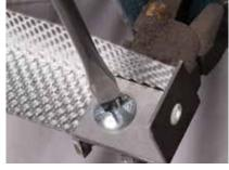
Gypframe FEA1 Steel Angle or Gypframe MF8 Strap Hanger is secured to Gypframe MF12 Soffit Cleats with Gypframe MF11 Nuts and Bolts to form hangers.
