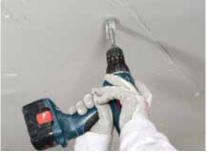
Mark the position required for the suspension points and fasten the CasoLine MF12 Soffit Cleats to soffit.
