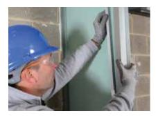
Gypframe 'I' Studs or Gypframe Tabbed 'I' Studs are friction fitted into the channels at 600mm required centres. Gyproc CoreBoard or 20mm Glasroc F FIRECASE is fitted between the studs on the shaft side, and held in place with appropriate Gypframe Retaining Channels. Door openings are formed to the **ShaftWall** Access Door Details.
