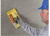
The final coat is ruled to an even surface and lightly scratched to form a key for Gyproc Finish Plasters.
