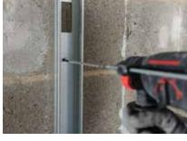
Gypframe 'C' Studs are suitably fixed to abutments and door openings.
