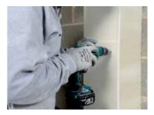
For four-sided protection to steel columns, Glasroc F FIRECASE boards are positioned and fixed board to board using Glasroc  $\mathsf{F}\xspace{\mathsf{Firecase}}$ Screws.
