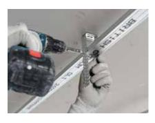
Gypframe GL1 Lining Channels are located into the perimeter track and each leg of the Gypframe GL2, GL9 or GL12 Brackets are screw-fixed to the Gypframe GL1 Lining Channels with Gyproc Wafer Head Drywall Screws.
