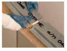
Gypframe SIF Floor Channels are located centrally over the joists. They must not be fixed to the joists.
