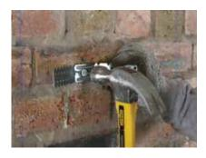
Vertical lines are marked on the wall at 600mm intervals to indicate Gypframe GL2 or GL9 Bracket fixing centres. Horizontal lines are marked at 800mm centres to determine individual bracket positions. Gypframe Brackets are then fixed into position.
