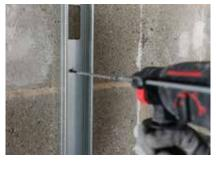
Gypframe 'C' Studs are suitably fixed to abutments.
