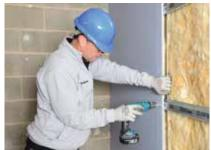
Gyproc plasterboards are fixed with Gyproc Drywall Screws to the Gypframe RB1 Resilient Bars with all joints staggered. Where Gyproc Plank is required as an inner layer, it is fixed horizontally to the Gypframe RB1 Resilient Bars at each bar position.
