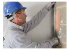
Gyproc plaster Angle Bead or Gyproc plaster Stop Bead is fixed to the background by embedding in the undercoat plaster.
