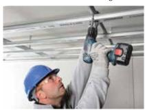
Gypframe MF5 Ceiling Sections are fixed to the underside of the Gypframe MF7 Primary Support Channels to form a grid with Gyproc Wafer Head Jack-Point Screws.
