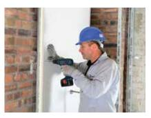
Gyproc plasterboards or thermal laminates are then fixed to all framing members with Gyproc Drywall Screws.
