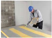
The fitting of Gypframe Skirting Plates over the bottom edge of the boards during installation provides a ground for subsequent skirting fixing.
