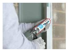
Pressurised shafts and service ducts are sealed using Gyproc Sealant. This is applied to all board-to-metal junctions.
