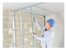
Gypframe studs are then friction fitted into the Gypframe Floor & Ceiling Channels at required centres.
