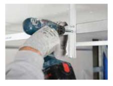
Gypframe MF7 Primary Support Channels are fixed to the hangers with Gyproc Wafer Head Jack-Point Screws, two per hanger.
