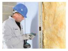
Gyproc plasterboards are then fixed to the Gypframe framework with Gyproc Drywall Screws and Gyproc Jack-Point Screws.
