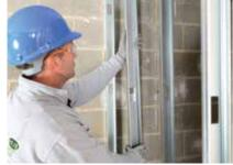
Gypframe 'C' Studs are suitably fixed to abutments in two rows.
