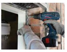
Gyproc Edge Bead can be fixed to window or door frames to provide edge protection to the reveal and soffit linings.
