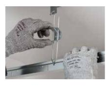
Use CasoLine QUICK-LOCK GRID Hangers to suspend the CasoLine QUICK-LOCK GRID 15/38 Main Tee.
