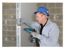
Gyproc DuraLine (and Gyproc SoundBloc inner layer if required) plasterboards are then fixed to the Gypframe framework with Gyproc Drywall Screws.
