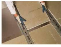
Gyproc Plank is cut neatly to fit between the channels.
