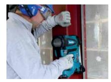
For two or three-sided beams or columns Gypframe GA2 Steel Angle is located to both sides of the wall / soffit flange and secured using appropriate fixings.
