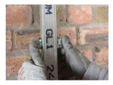
The protruding Gypframe Bracket legs are bent back to sit clear of the Gypframe GL1 Lining Channel face. At internal angles, a Gypframe GL1 Lining Channel is positioned tight into the corner to provide support for the lining.
