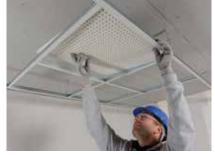
**CasoLine QUICK-LOCK GRID** is self-squaring, so with the CasoLine QUICK-LOCK GRID 15/38 Cross Tee in place to form the grid, tiles can be easily laid into place.
