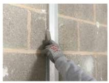
The board edge positions are marked on the wall, and Gyproc Plasterboard Compound is applied to the wall in dabs to support the boards.
