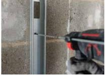
Gypframe Studs are suitably fixed to abutments.
