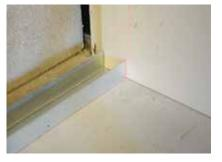
Gypframe Floor & Ceiling Channels are suitably fixed to the floor and soffit. Gypframe 'C' Studs are suitably fixed to openings and abutments.
