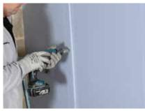
Gyproc plasterboards are then fixed to the Gypframe framework with Gyproc Drywall Screws.
