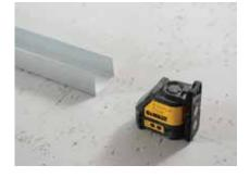
Gypframe Deep Flange or Extra Deep Flange Floor & Ceiling Channels are suitably fixed to the floor and soffit.
