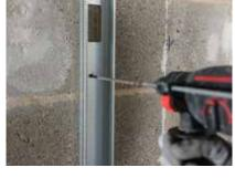
Gypframe Studs are suitably fixed to abutments.
