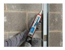
The perimeter of the partition is then sealed with Gyproc Sealant except where Gypframe RB1 Resilent Bars are to be installed on that side. Where Gypframe RB1 Resilient Bars are to be installed, the Gyproc Sealant is applied to the perimeter of the first layer of board.
