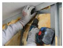
Isover Acoustic Roll is added to the partition cavity.
