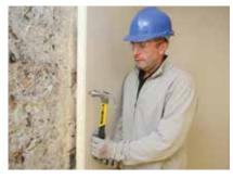
When installing Gyproc ThermaLine laminate in the **DriLyner n** system, insert two Gyproc Nailable Plugs at mid height after dabs have set, as secondary mechanical fixings.
