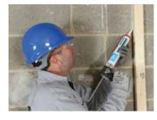
The perimeter of the partition is sealed on both sides with Gyproc Sealant.
