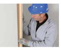
At reveals and external angles the lining is run past the corner and the insulating backing is cut back so as to form a neat junction with the reveal board or wall lining.
