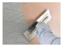
Once the Gyproc undercoat plaster has set, Gyproc Finish Plaster is applied with firm pressure, built out to the required thickness in two applications and trowelled to a smooth matt finish. In some circumstances it may be necessary to control the suction with Gyproc GypPrime. Good site practice should be followed, as outlined in BS EN 13914 - 2 Design considerations and essential principles for internal plastering.
