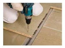
Flooring is laid across the Gypframe SIF Floor Channels and screw-fixed through the Gyproc Plank to the channel flange on one side only, using Gypframe SIF5 Floor Screws. It is important to ensure that no fixings are allowed to connect the Gypframe SIF Floor Channels to the joists.
