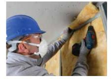
Isover Acoustic Roll insulation is added to the partition cavity for optimal acoustic performance.
