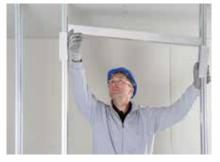
Door openings are constructed to the Heavy and Severe Door Duty Rating detail.
