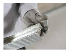
Gypframe SC1 or SC2 Spacer Clips are inserted to the top and bottom of the Gypframe 60 I 70 or 92 I 90 'I' Studs respectively.
