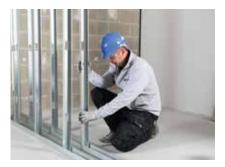
Gypframe 'C' Studs are then friction fitted into the Gypframe Floor & Ceiling Channels at the required centres. Door openings are constructed to the Heavy and Severe Duty Rating door detail.
