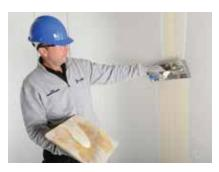
Two or three further applications of jointing compound are trowel applied, each feathered out beyond the previous application. An equal number of applications are made to spot screw heads. Once dried, the joint treatment is sanded as necessary to achieve a smooth surface.
