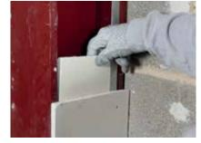
Additional layers of Glasroc F FIRECASE are fixed as before, with staggered joints. For single layer steel beam encasements, additional strips of Glasroc F FIRECASE are installed behind the ends of the facia board-ends so as to seal the joints.
