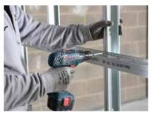
Gypframe RB1 Resilient Bars are fixed transverse to the stud framing. Gypframe RB1 Resilient Bars are joined by nesting them together over a Gypframe 'C' Stud using Gyproc Wafer Head Drywall Screws. Gypframe RB1 Resilient Bars are normally fixed with the base flange on the top side, with the exception of the uppermost bar, which is fixed base flange down to provide board fixing at the head.
