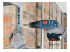
Openings and reveals are formed with Gypframe GL1 Lining Channels and Gypframe GL8 Track.
