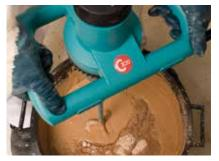
Gyproc plasters should be mixed by adding to clean water and using clean mixing equipment. Contamination from previous mixes must be avoided as this can adversely affect the setting time and strength.
