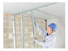
Gypframe 'C' Studs are fitted vertically to a friction-fit within the channel sections, to form the framework. Studs are fitted to all face the same way.
