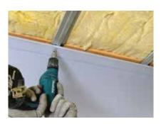
When fixing boards, care must be taken to ensure that the plasterboard fixing screws do not make contact with the joists.
