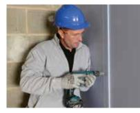
Gyproc plasterboards are screw-fixed to all timber supports with Gyproc Drywall Screws, or to the Gypframe RB1 Resilient Bars with Gyproc Drywall Screws.
