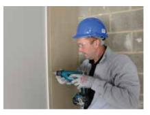
Rigidur boards are then fixed as the outer layer to all Gypframe framing members with Rigidur Screws.
