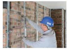
Gypframe GL1 Lining Channels are friction-fitted into the track, extending if required.
