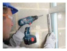
Gypframe RB1 Resilient Bars are installed vertically to abutment and door studs to accept perimeter fixings for the Gyproc plasterboard linings.
