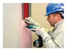
Boards are cut to width and fixed to all framing members using Gyproc Drywall Screws.
