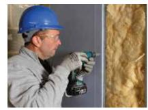
Gyproc SoundBloc plasterboards are then screw fixed to alternate Gypframe 'I' Studs and other framing members with Gyproc Jack-Point Screws.
