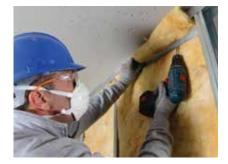
Isover acoustic insulation can also be added to the partition cavity for increased acoustic performance.
