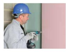
Gyproc plasterboard or Glasroc F FIRECASE are then fixed to the Gypframe framework with Gyproc Drywall Screws or Gyproc Jack-Point Screws.
