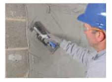
Once the correct Gyproc plaster has been selected to suit the background suction and surface texture, the plaster is applied in maximum 8mm coats. Each coat is allowed to set before applying the next.
