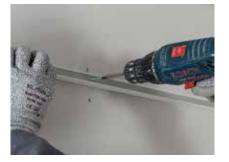
Measure and mark the required ceiling height, then fix the CasoLine QUICK-LOCK GRID WA02 Wall Angle or WA03 Wall Angle around the perimeter of the ceiling area to suit.
