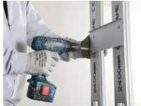
The two frameworks are braced with Gypframe 99 FC 50 Fixing Channel attached to the Gypframe 'C' Studs with Gyproc Wafer Head Drywall Screws, two screws per junction.
