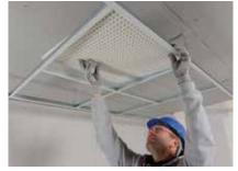
**CasoLine QUICK-LOCK GRID** is self-squaring, so with the CasoLine QUICK-LOCK GRID 24/38 Cross Tee in place to form the grid, tiles can be easily laid into place.
