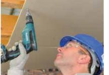
Gyproc plasterboards can be fixed directly to the underside of timber joists. Timber noggings are fitted, where required, between joists at room perimeters to support board edges. Noggings may also be required to support board edges in the field of the boards. Plasterboards are fixed to timber supports using Gyproc Drywall Screws.
