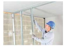
Gypframe Studs are then friction fitted into the Gypframe Floor & Ceiling Channels at the required centres.
