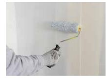
Gyproc Drywall Primer or Gyproc Drywall Sealer is applied to the entire board surface and jointed areas, to prepare the lining for final decorative treatment.
