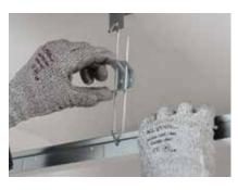
Use CasoLine QUICK-LOCK GRID Hangers to suspend the CasoLine QUICK-LOCK GRID 24/38 Main Tee.
