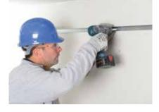
Gypframe MF6 Perimeter Channels are fixed to the perimeter walls at 600mm centres.
