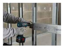
M&E services can be located within the partition cavity. Care should be taken to prevent bridging, for example socket boxes making contact with the opposing studs.
