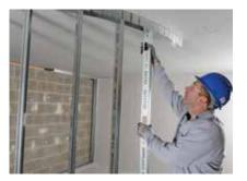
Gypframe studs are fitted and fixed into the Gypframe 72 EDCL 80 CurveLyner Channels at the required centres. If a deflection head is required, the studs should not be fixed into the head channel and alternative temporary support may be required to stabilise the stud at the head whilst boarding proceeds.
