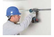
Gypframe GL8 Track is fixed at the perimeter of the room with the longer leg at the bottom.
