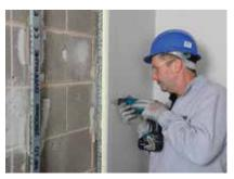
A continuous fillet / ribbon of Gyproc Plasterboard Compound is applied to the wall perimeter and around all services and openings as board fixing proceeds. This is particularly important if the lining is designed to act as an air barrier to achieve building airtightness. Boards are screw-fixed to all Gypframe MF10 Channel supports. Screw lengths should be selected to avoid contact with the masonry background.
