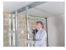
Gypframe 92 S 10 'C' Studs are then friction fitted into the Gypframe Channels at the required centres, and door openings are constructed to the Heavy and Severe Duty Rating door detail.
