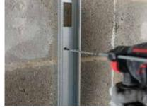
Gypframe 'C' Studs are suitably fixed to abutments and at openings.
