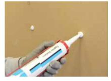
The wall is marked with lines at 900mm or 1200mm centres to indicate board positioning. Drylining is commenced from a window / door reveal or internal angle. Gyproc Sealant is gun-applied to the wall, or the back of the board, in blobs at 300mm centres.
