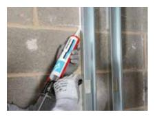
Gyproc Sealant is applied to the frame perimeters to seal airpaths.
