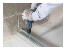
The appropriate Gypframe channels, are suitably fixed to the floor and soffit of the structure. Gyproc FireStrip is used on the channel at the soffit.
