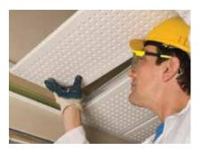
Gyptone Planks are cut to fit on the lower flange of the CasoLine QUICK-LOCK GRID Shadowline Moulding CLSM04.
