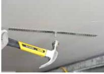
Gypframe GL2, GL9 or GL12 Brackets are fixed to the sofit at the required centres.
