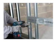
Mechanical and electrical services can be located within the partition cavity.
