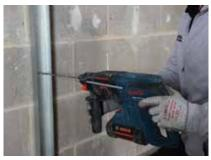
Gypframe Starter Channels are suitably fixed to vertical abutments. The perimeter of the partition is sealed with Gyproc Sealant.
