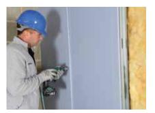
When applying muliple layers of board, ensure that all board joints are staggered on both sides of the partition.
