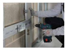
If specified, Isover acoustic insulation is fitted between studs. Electrical and other services are normally installed at the frame erection stage. Horizontal runs are fixed to the background or can be routed through cut-outs in the studs.
