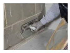
A continuous fillet / ribbon of Gyproc Plasterboard Compound is applied to the wall perimeter and around all services and openings as board fixing proceeds. This is particularly important if the lining is designed to act as an air barrier to achieve building airtightness.
