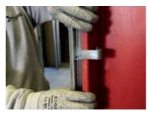
Gypframe GL1 Lining Channels are located over the clips to form the steel framework.
