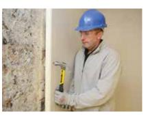
When installing Gyproc ThermaLine laminates in the **DriLyner RF** system, insert two Gyproc Nailable Plugs at mid height after Gyproc Sealant has set, as secondary mechanical fixings.
