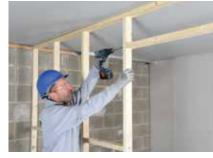
Door openings are formed by fixing full height timber studs to each side, together with a timber head piece. Door casings are then fixed to the timber ground. Additional framing is installed as required to support heavy fixtures.
