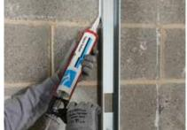
The perimeter of the partition is then sealed on both sides with Gyproc Sealant.
