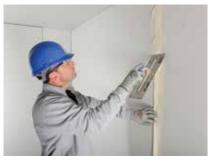
For external corners Gyproc Corner Tapes are bedded with a Gyproc setting compound.
