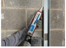
The perimeter of the partition is then sealed on both sides with Gyproc Sealant.
