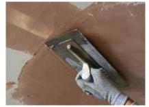
For best results Gyproc plaster is applied with firm pressure, built out to the required thickness in two applications and trowelled to a smooth matt finish. Good site practice should be followed, as outlined in BS EN 13914 - 2: Design Considerations and Essential Principles for Internal Plastering.
