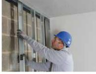
Gypframe 'I' Studs are friction-fitted vertically at the required centres within the channel sections to form the framework. Additional framing is installed as required to support heavy fixtures.
