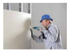
Gyproc plasterboards or Glasroc specialist boards are then fixed to the Gypframe framework with Gyproc Drywall or Jack-Point Screws. The plasterboards are fixed horizontally, with all joints staggered. Additional studs may be required where multiple layers are specified to account for the difference that arises between inner and outer radii.
